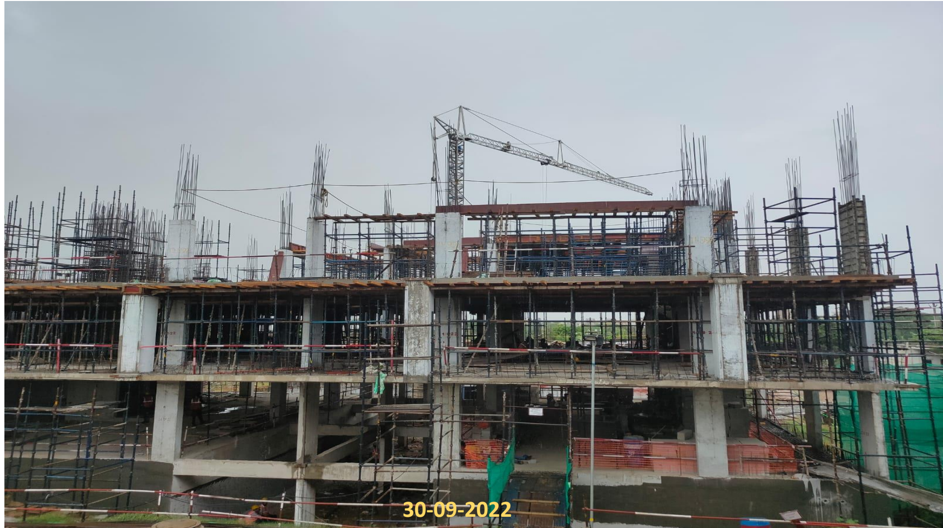
D7 - 1,2,3 – Terrace roof in progress
