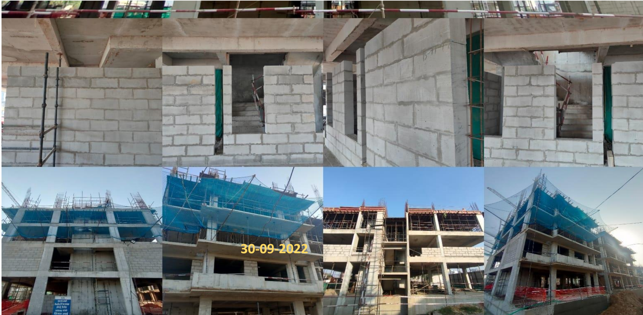
Blockwork in Basements of D block
